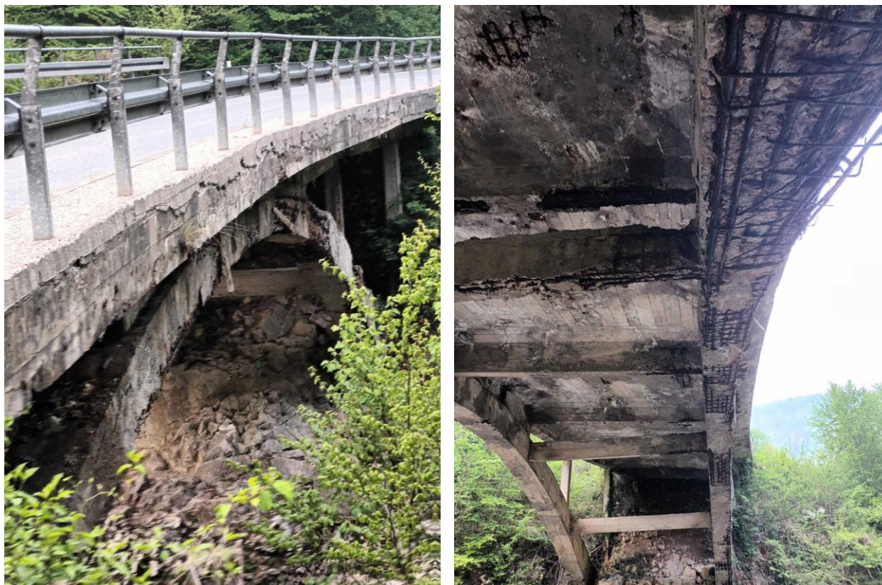
Figure 5: Drinjaca River Bridge – current state
